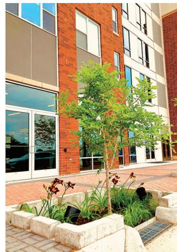
*Stormwater planter box in Coralville, Iowa. This practice is coupled with underground rock chambers to treat stormwater runoff from the roadway and sidewalks.*
