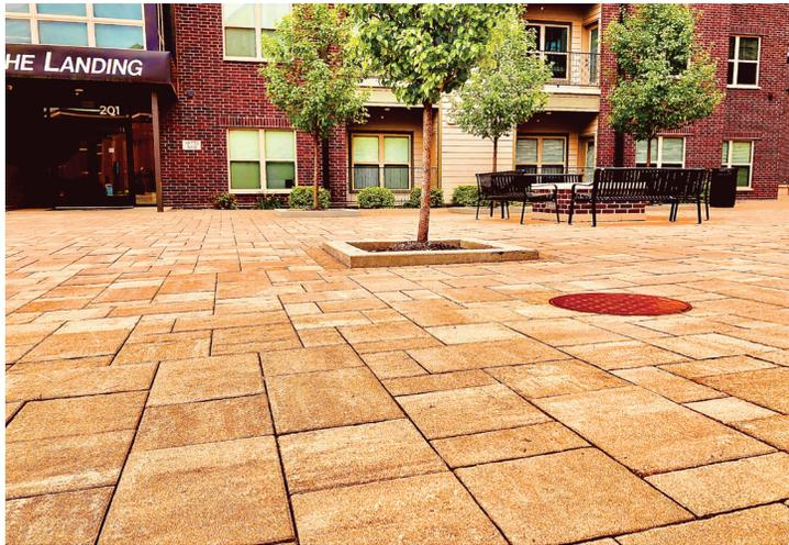
*Porous paving patio in Coralville, Iowa. This practice is coupled with tree infiltration trenches which clean and infiltrate stormwater from the adjacent roof.*
