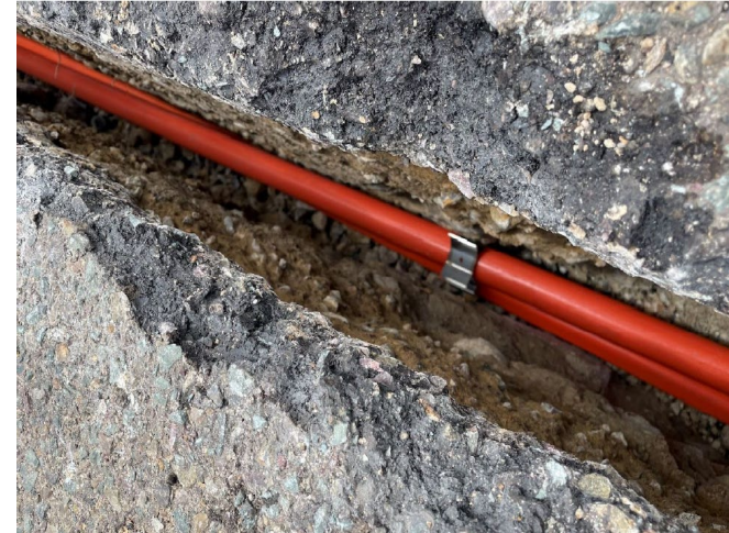
Cobble difficult to Maintain 2 ½" width and uniform edges, also broke equipment
